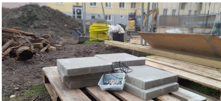
Figure 7: Construction area in Malmö Östervärn
