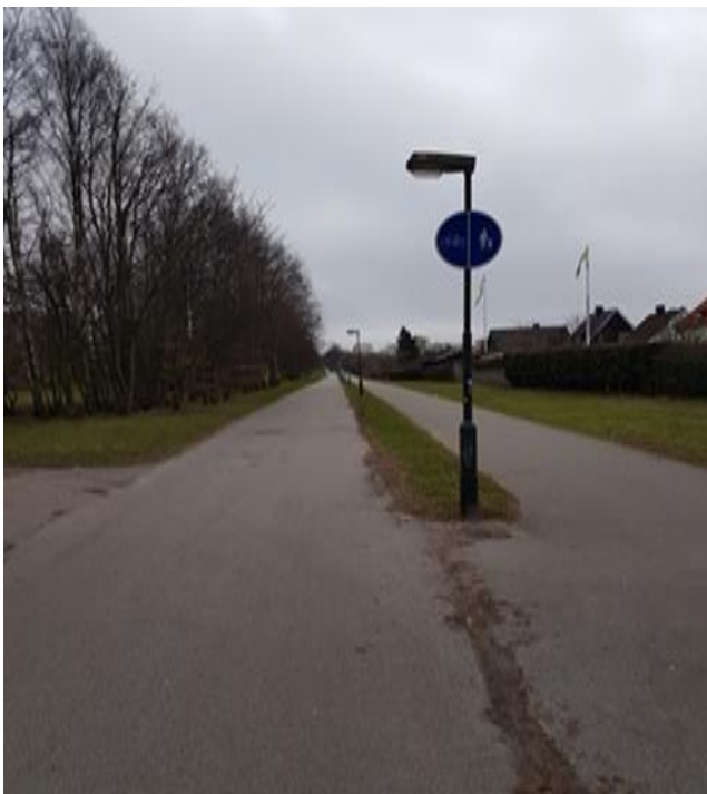
Figure 5 Picture of the hot spot part of the bike path
