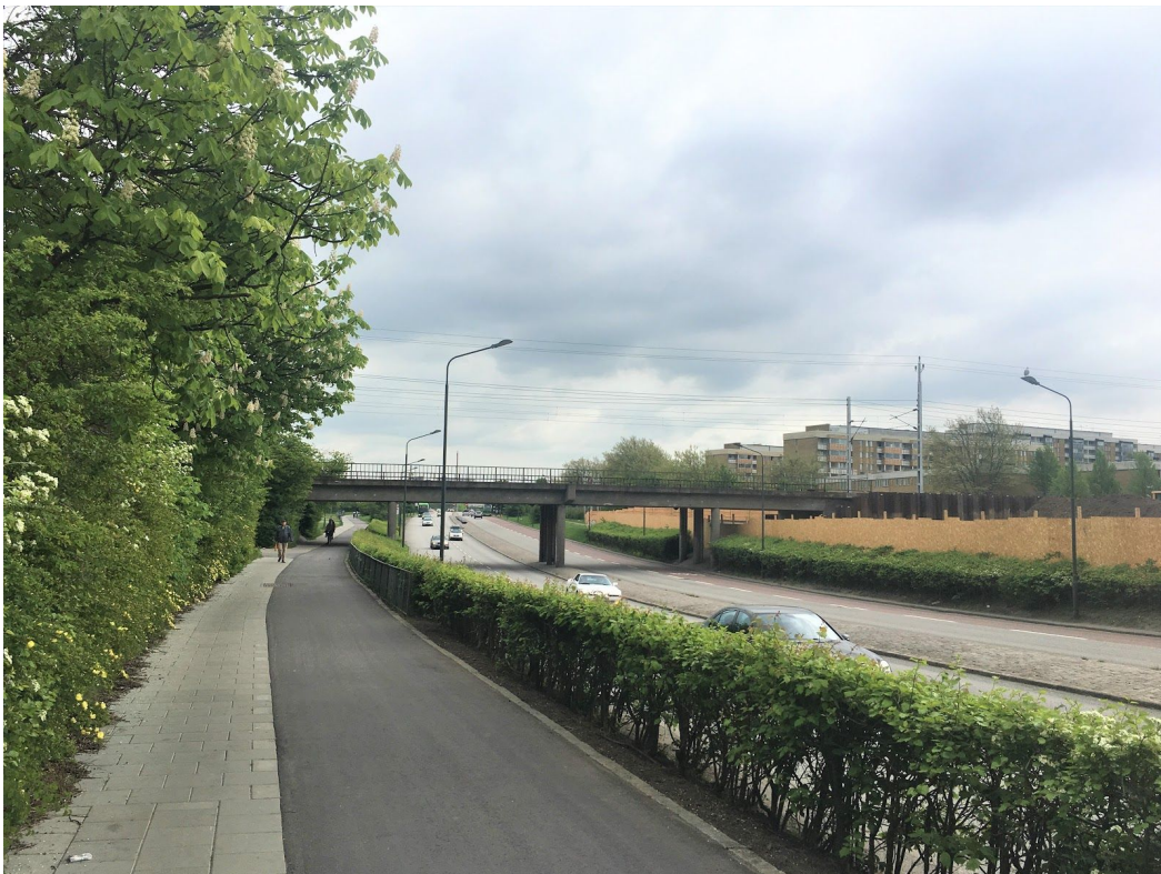
Figure 5. Photo of the bridge over Amiralsgatan
