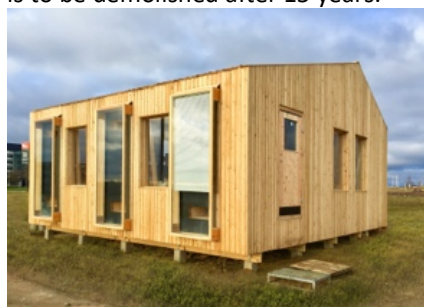
Fig. (1) The refugee house after construction.
